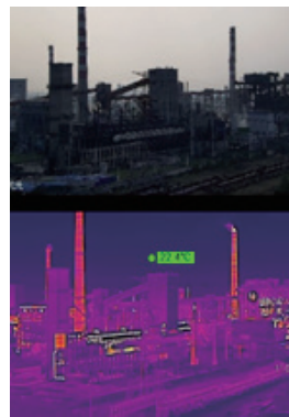
Industrial Park Monitoring
